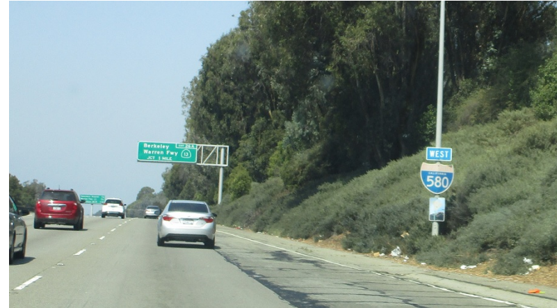
Missing paint, dirt
