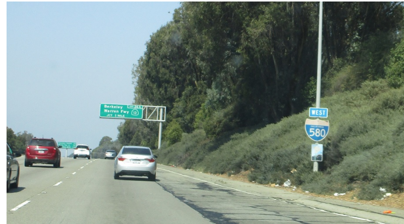
Missing paint, dirt
